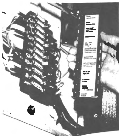
Fig. K:26 Fuse block
