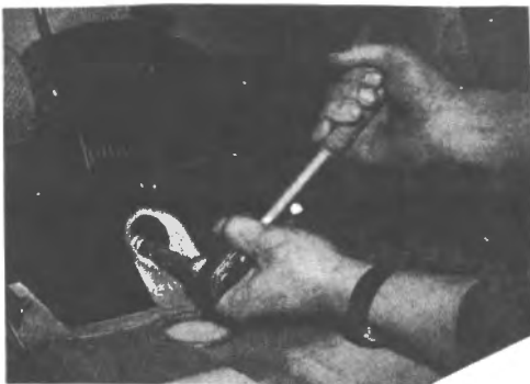
Fig. F:27 Releasing the rear engine mounting centre bolt.
